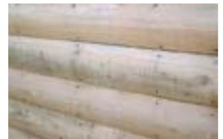
Dark colored streaks caused by metallic tannates. *Oxcon* solution will also remove rust stains caused by nails, screws and fasteners.
